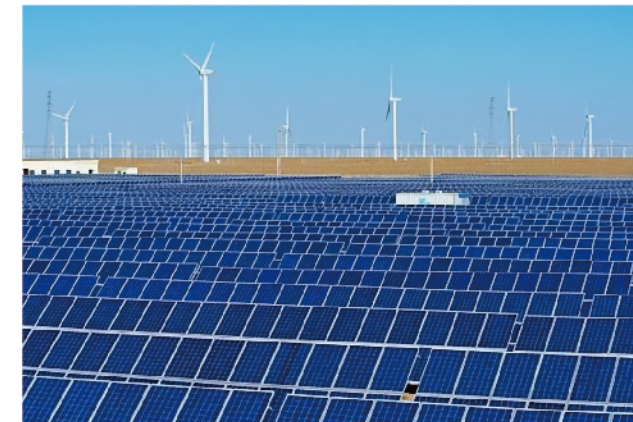
Integrated Energy System
